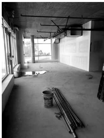
The first floor, looking toward PC office.
