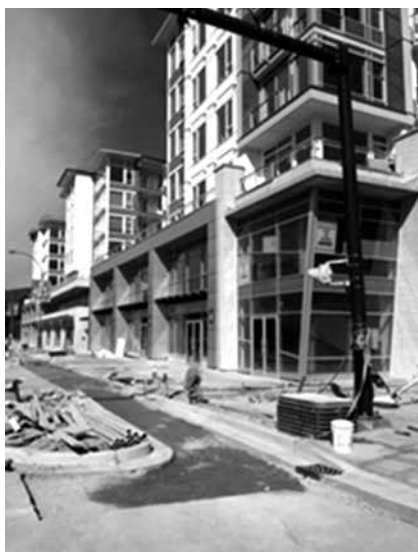
New building on the block!
